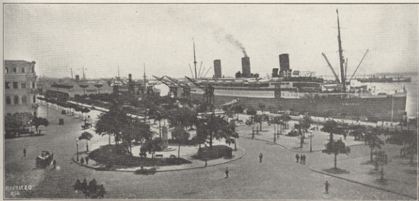
THE CAES DO PORTO AT RIO DE JANEIRO, SHOWING SOME OF THE ELECTRIC CRANES
