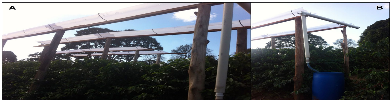
Figure 1: The infrastructure of the rain exclusion system: translucent polyethylene trough above the coffee planting lines. (A) Channeling rainwater from the gutter to a PVC pipe (B) PVC pipe directed to a 200-liter reservoir.
